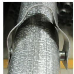
Fig 5: Un-secured Clamp
